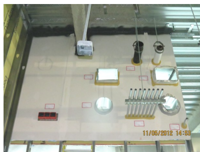
Good example of a fire stopping and head-of-wall mock-up
